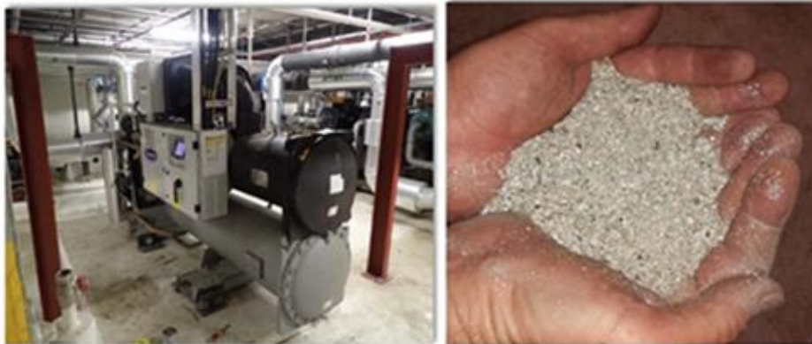
Existing Scales dislodged from Cooling H 2 O System during DCI operation
