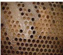
A badly scaled/fouled heat exchanger
